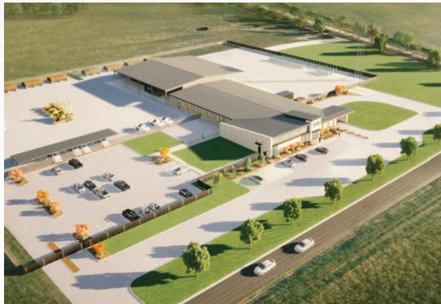
The co-op’s new headquarters at 2201 FM 87 in Bonham will benefit members. It will have a drive-thru for ease and convenience.
